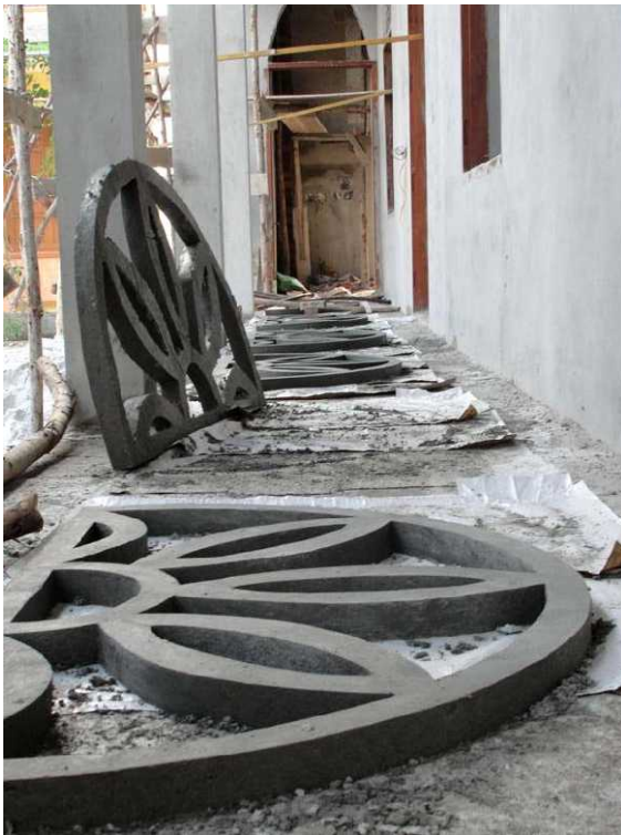
2 April. Site cast concrete vents drying off and being fitted above windows.
