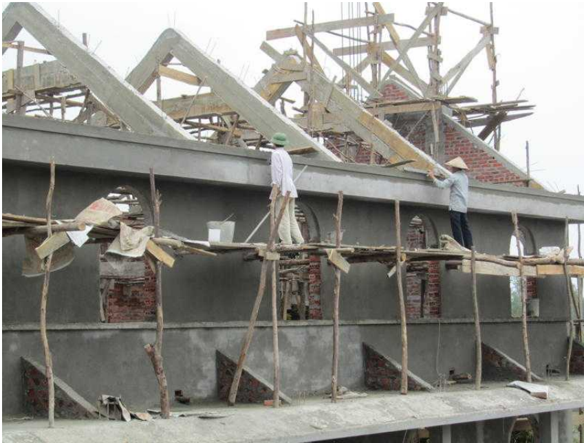
12 March 2011. Detail of roof beams and scaffold.
