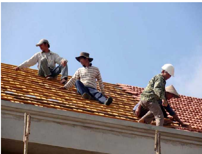
23 March roof framing and tiling.
