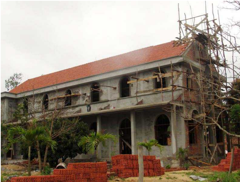
Completion roof tiling.
