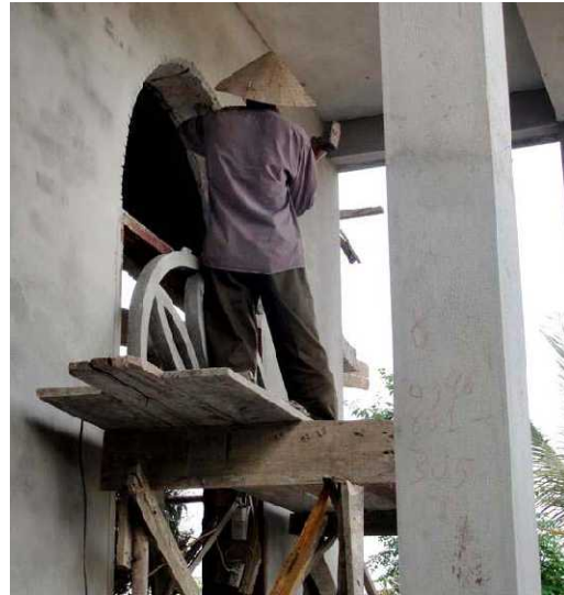
2 April. Site cast concrete vents drying off and being fitted above windows.
