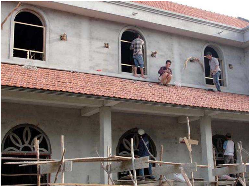
2 April window framing in progress.
