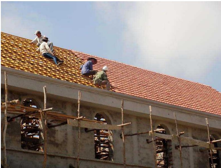
23 rd March roof tiling.
