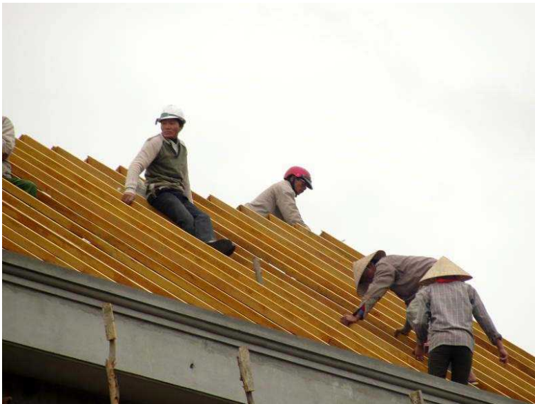
23 March roof framing.
