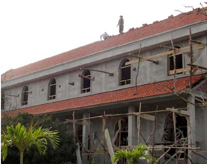
2 April. Ridge tiling being completed.
