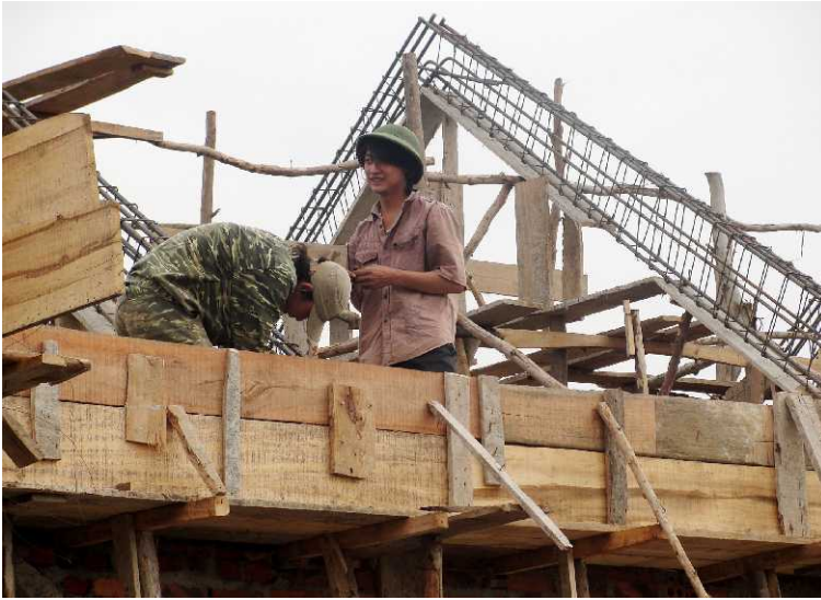
26 th Feb 2011. Concrete roof frame forming.
