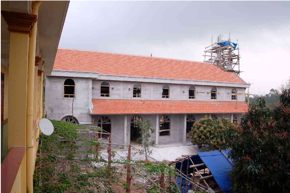
Stage 1 close to lock-up stage.
