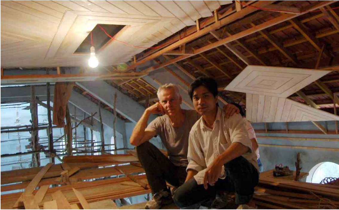
Hole for fluorescent office light is in the ceiling, some 10m above the floor.
