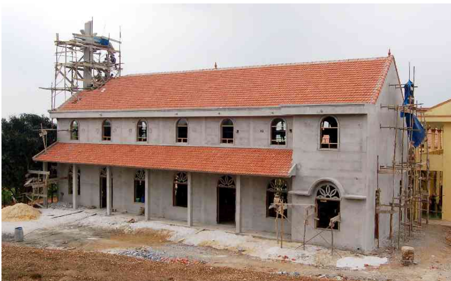
Stage 1 close to lock-up stage.
