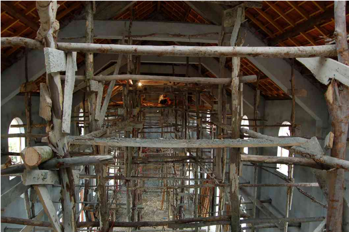
Vietnamese scaffolding held together with tie wire and nails but still seems to work.
