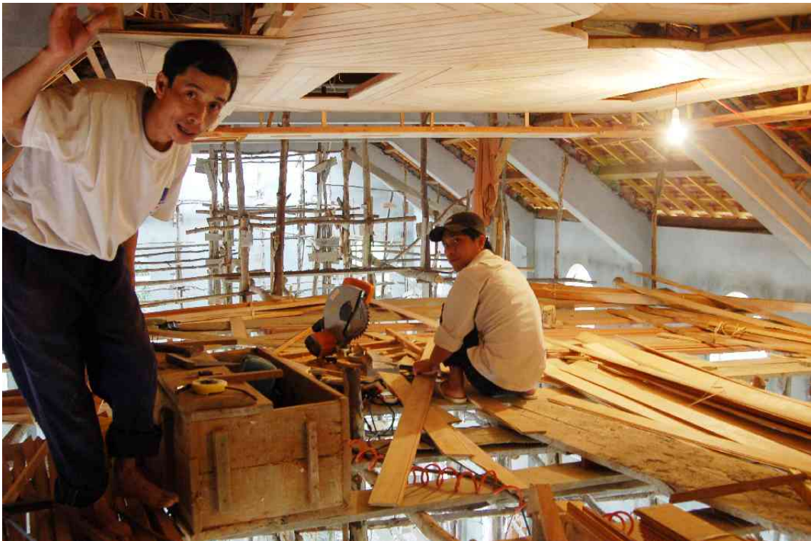
Ceiling workers on scaffold.
