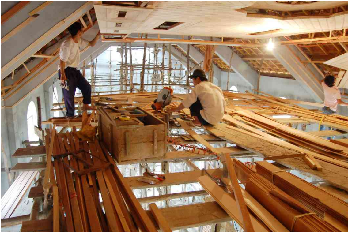
Ceiling workers on scaffold.
